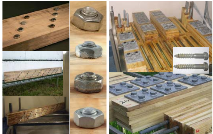
Figure 4: Samples acetylated Radiata Pine from the corrosion test: left different types of corrosion protection systems; right types of fastener to be used in the bridges, incl. glued-in rods
