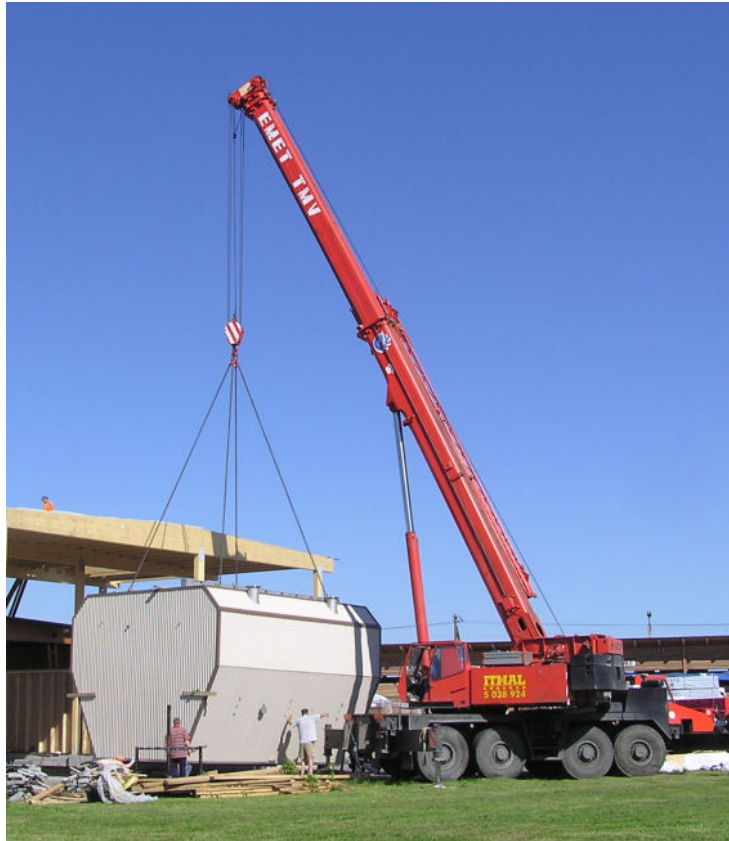
Figure 2: Installation of a 12 m 3 Stellac Kiln
