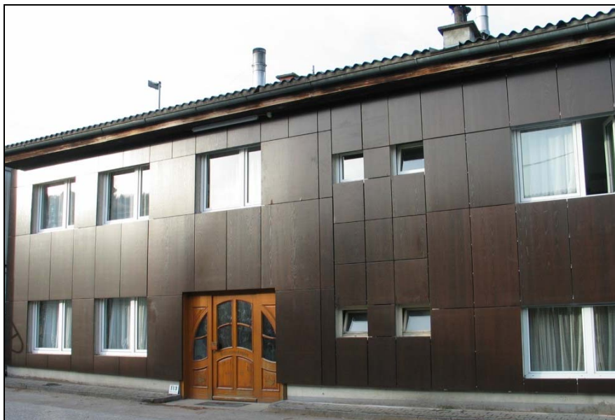
Figure 7: Office Façade at Mitteramskogler
