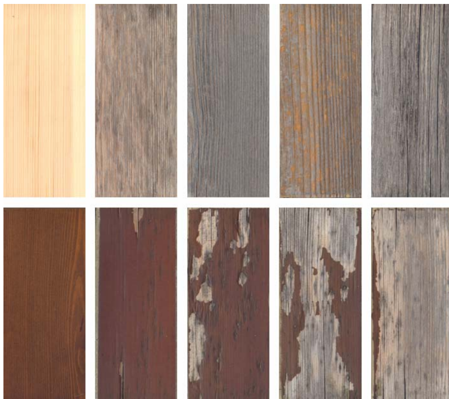
Figure 1. Appearance changes to wooden facades due to weathering
