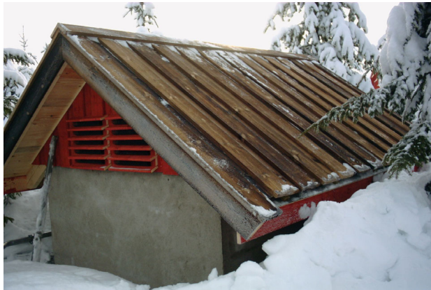
Figure 6: Roof made of pine VisorWood.
