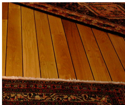
Figure 10: Intermediate layers of beech Kebony Dark In shipdeck-style parquet flooring.
