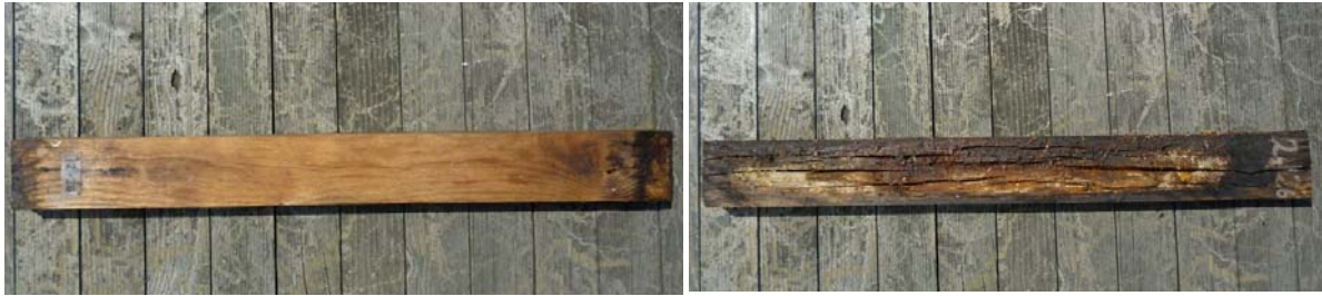
Figure 2: Appearance of TMT ash stakes from double layer test, lower layer, after 6 years: left: lower side of the stake (facing down to the ground) without decay right: upper side (facing to the interstice between the layers) with heavy decay
