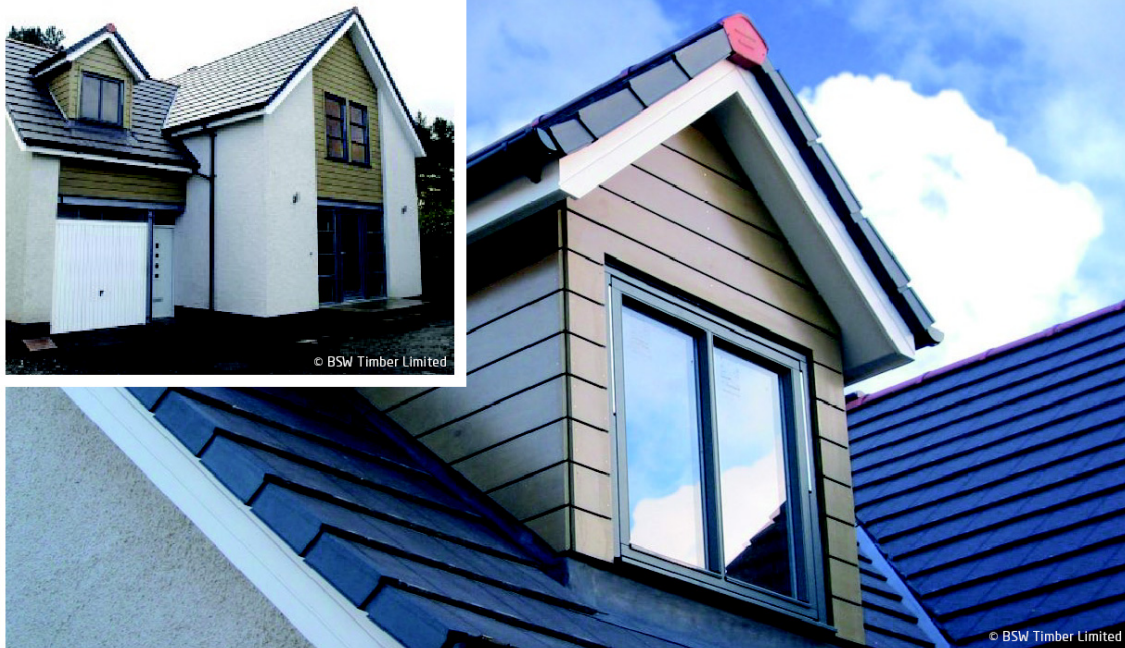
Figure 4: Cladding project Fife (UK)
