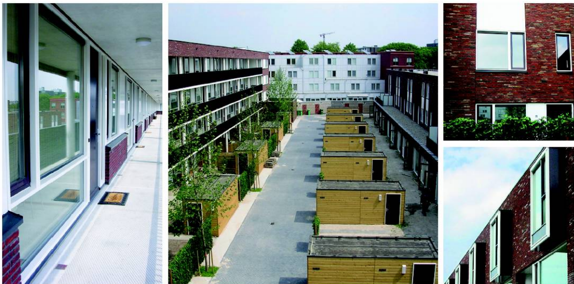
Figure 3: Joinery project Den Haag (NL)
