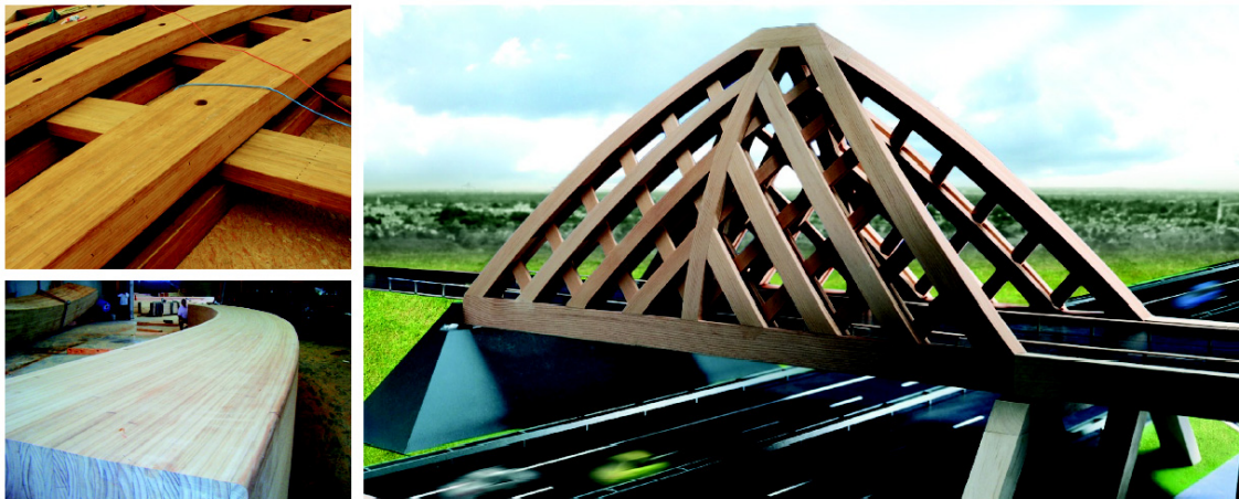
Figure 5: Accoya® bridge Sneek (NL)
