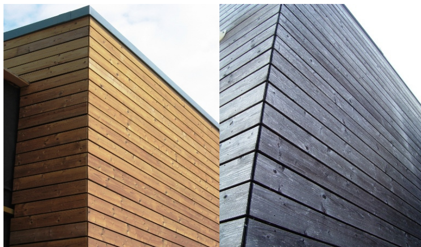
Figure 3. Broughton Fields Primary School, UK. In June 2004 (left) and in June 2008 (right).
