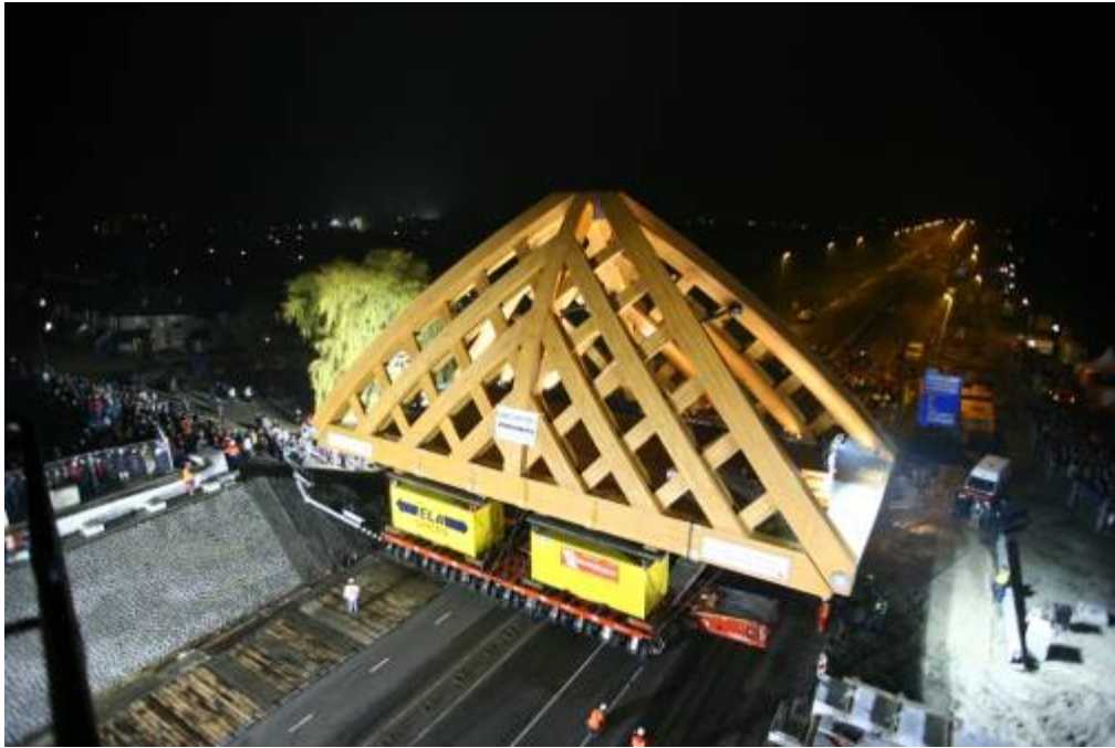
Figure 6: Transportation of the bridge to its final location over the high way A7 at Sneek
