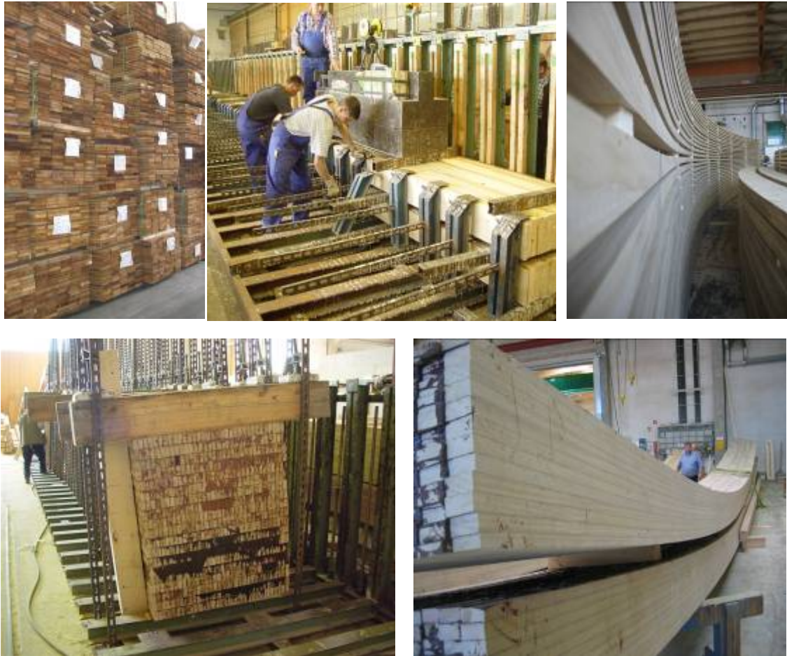
Figure 3: Two step lamination at Schaffitzel; For constructional reasons the wood is laminated in two phases. The acetylated planks are first machined into beams of 1.08m height(photo's above) which are rip-sawed into 60mm thick planks with a width of 1.08 metres. Then they are glued in another direction and formed into straight, curved and twisted beams measuring 1.08 by 1.40 metres (photo's below)
