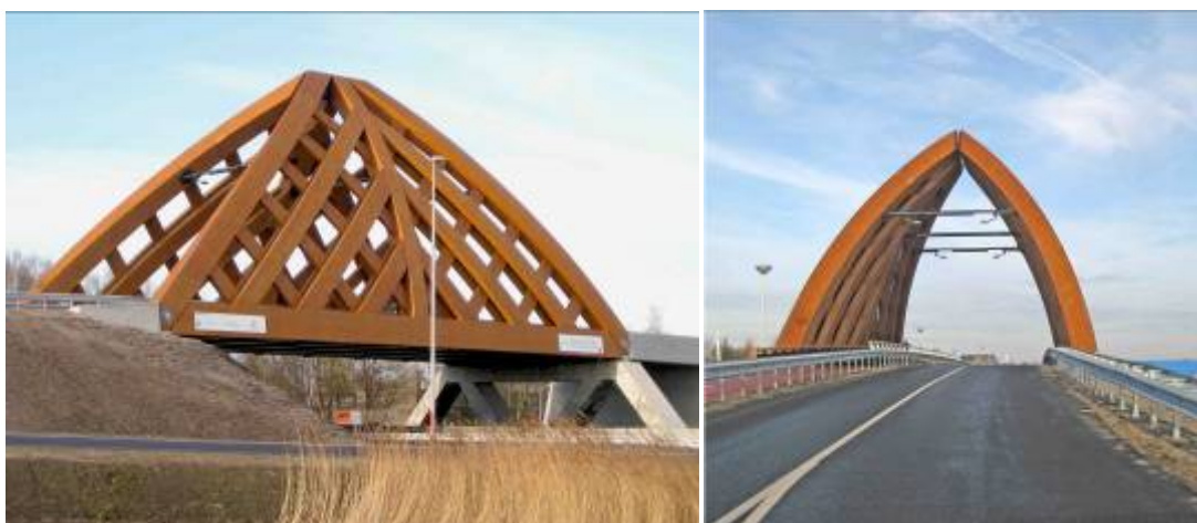
Figure 1: The timber traffic bridge made of Accoya ® wood
