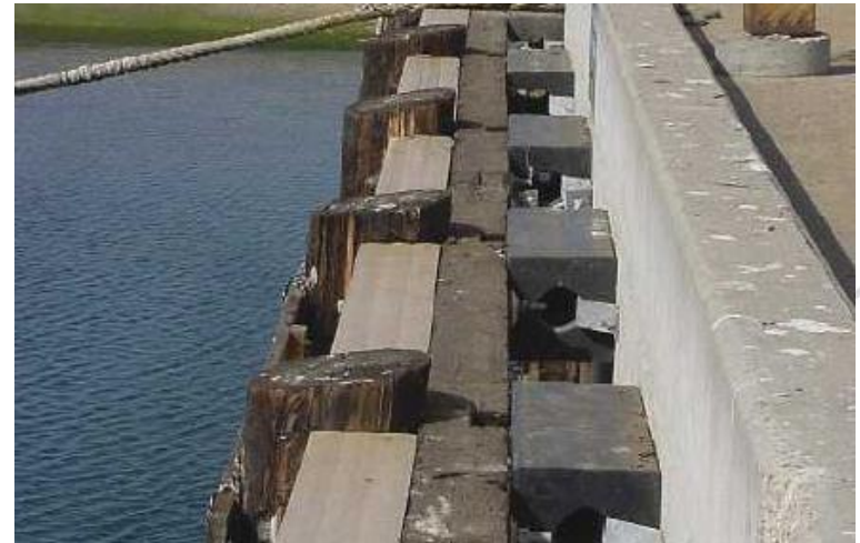
WPC Chock members in trials, Port Hueneme, California Source: Smith and Wolcott (2006) Forest Products Journal 56(3):4-11
