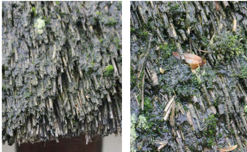
Figure 2: Decay and growth of mosses and algae on reed in the eaves on the North side of the building.
