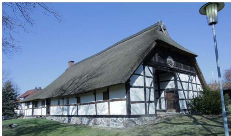
Figure 1: Museum building with cold roof thatched with reed ( Phragmites communis ) in Bortfeld, Germany.
