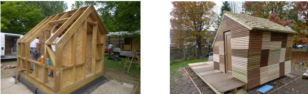
Fig. 1: Skeleton construction (left) and freshly installed façade (right) of the model house in Ljubljana.
