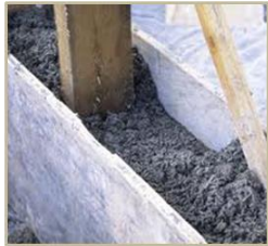
Shuttered HC wall
