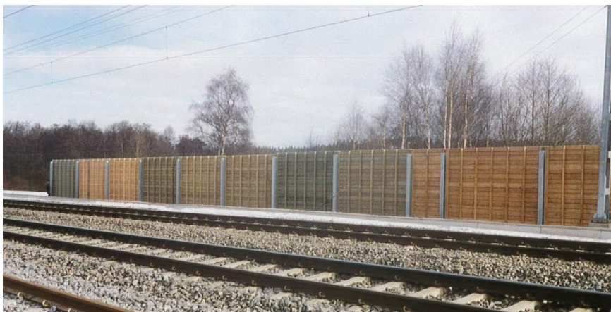
Figure 1: Noise barrier shortly after installation in March 1996
