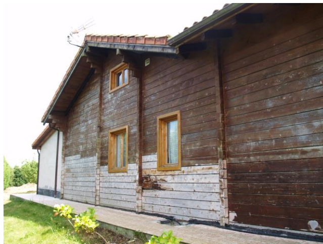
Figure 1: Fir wooden house located in Northern Spain.
