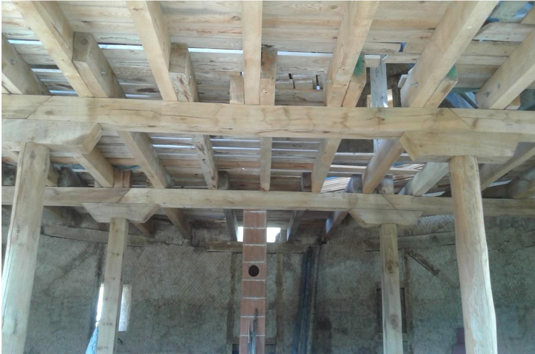
Fig. 7 The base is made of stone, without concrete, but with a wooden construction
