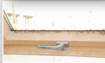
on the interior side moisture condensation mould grow decay
