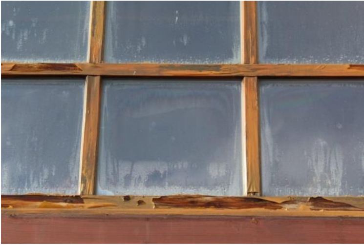
on the interior side moisture condensation mould grow decay
