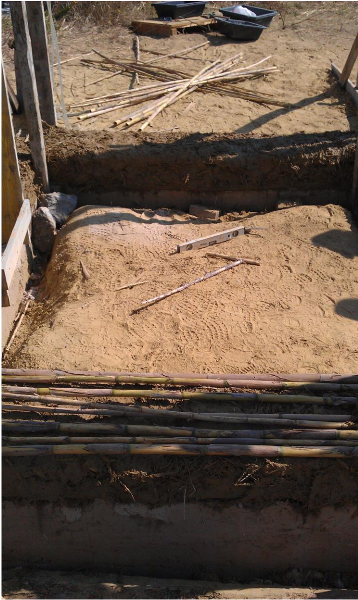
Successive layers of earth-reed fiber mortar and layers of reeds
