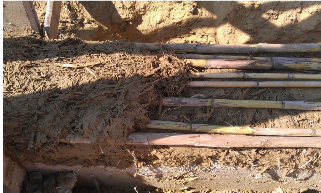
Successive layers of earth-reed fiber mortar and layers of reeds
