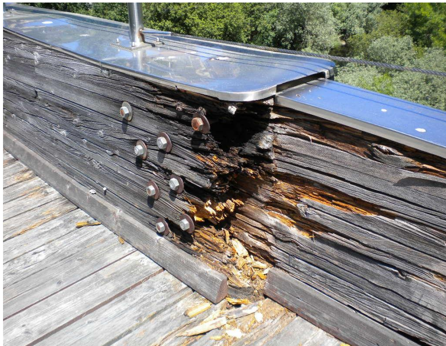
Spruce Bridges in North Spain with severe decays (12 years)
