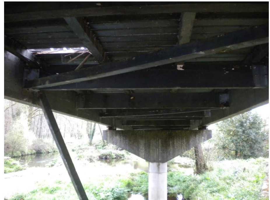
Spruce Bridges in North Spain with severe decays (12 years)
