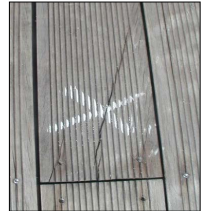
cracks due to slope of grain, ash TMT, photo: anonym
