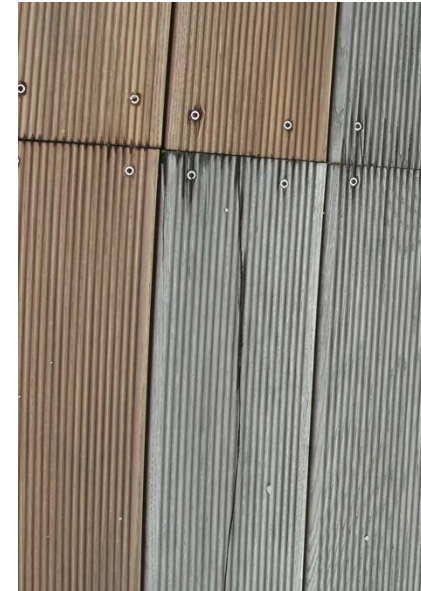
defective decking board, ash TMT, photo: anonym
