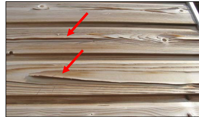
tangential delaminations, facade cladding, spruce TMT,
