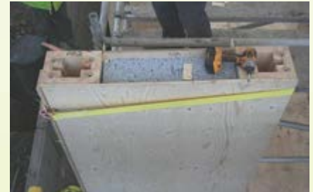
Construction panels can incorporate plywood, OSB, MDF and fibrous insulation. Picture courtesy Welsh School of Architecture
