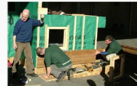
Training school on cladding installation (courtesy of WoodKnowledge Wales, UK)
