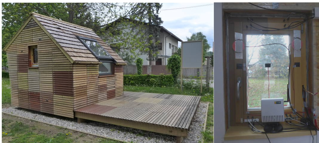
Figure 1: Test object with decking and façade elements after 18 months exposure and the installed window made of TM spruce (left half side) and spruce (right half side) profile with installed sensors for temperature, moisture and heat flux.
