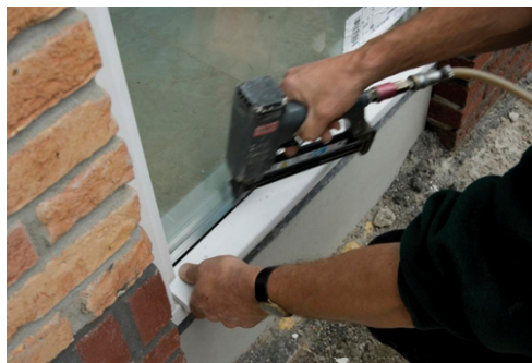
Figure 6: Typical on-site repair work of the 'weak' parts
