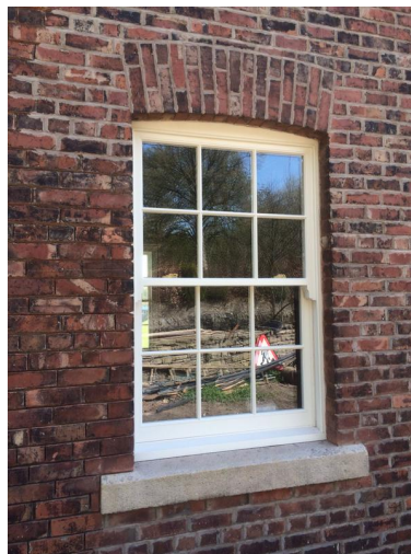
Figure 2: Accoya in a standard English sash window design
