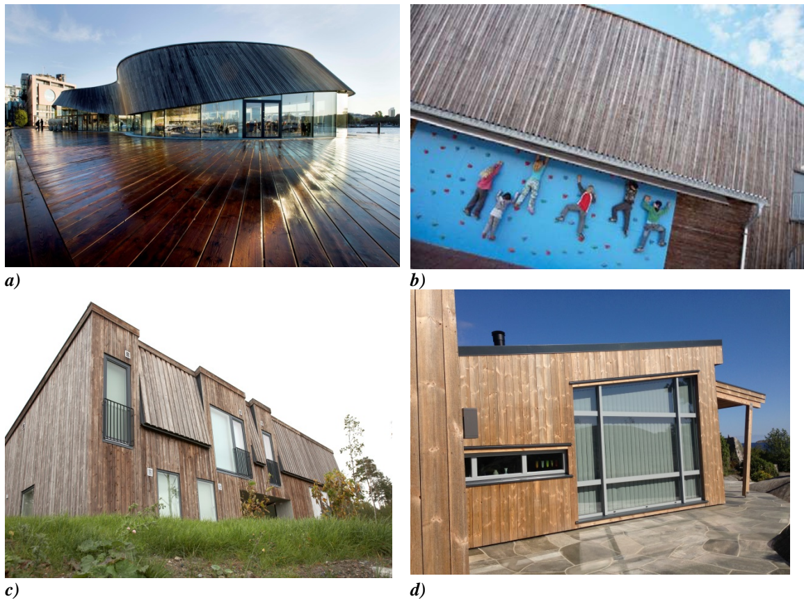
Figure 1: Home market; Kebony decking and cladding, mainly with Kebony scots pine. a) Onda restaurant in Oslo, b) Elementary school, c) Private home, d) Coast cottage
