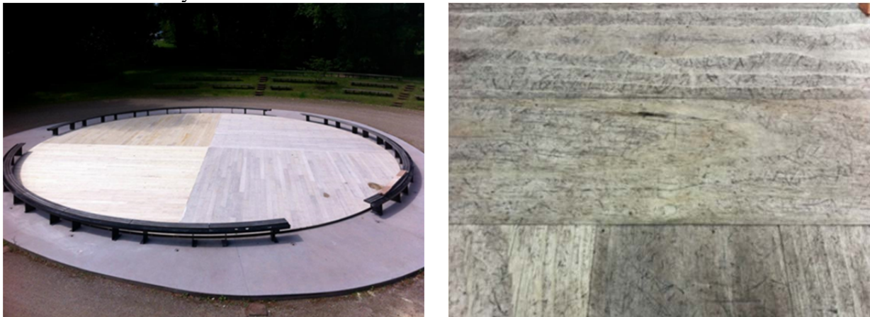
Figure 2: Overview of the exterior dance floor (left); Close up photo of the surface after 3 seasons before cleaning (right).
