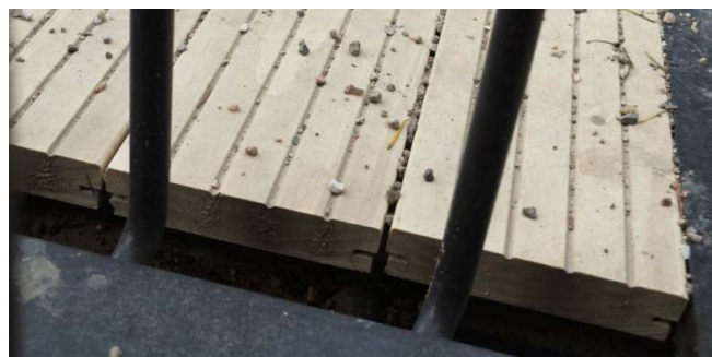
Figure 4: Accoya 34 x 198 mm bridge deck with hidden fasteners.
