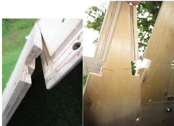
Figure 2: Under squinted scarf-joint between vertical details (on the left) and between horizontal details (on the right). (Montage and photo T.Teppand)
