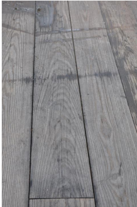
Figure 1: Cracks in decking board of thermally modified ash after two years in service (Hundhausen 2012)
