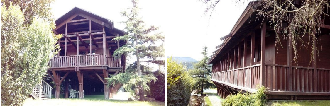
Figures 2 and 3: North facade and south-west facades.
