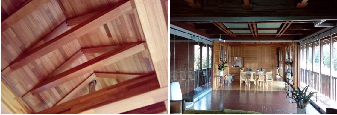
Figures 4 and 5: Roofing structure and interior all in glue lam Eucalyptus globulus..
