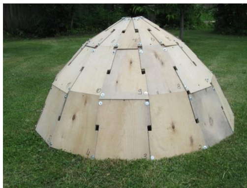
Figure 1: Semi-globe type dome-shell with self-locking under squinted scarf joints. (Montage and photo T.Teppand)
