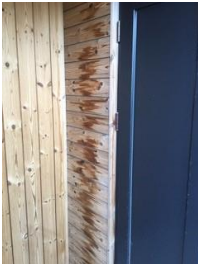
Figure 2: Colour change on cladding of thermally modified Scots pine cladding.
