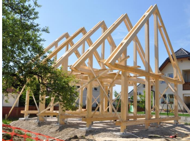
Figure 2: Timber frame structure.
