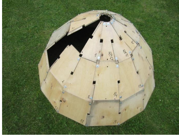
Figure 3: Mounting the dome-shell of details with prefabricated under squinted scarf-joints at the edges). (Montage and photo T.Teppand)
