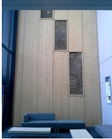
Figure 4: Truth windows in Gateway Building atrium.
