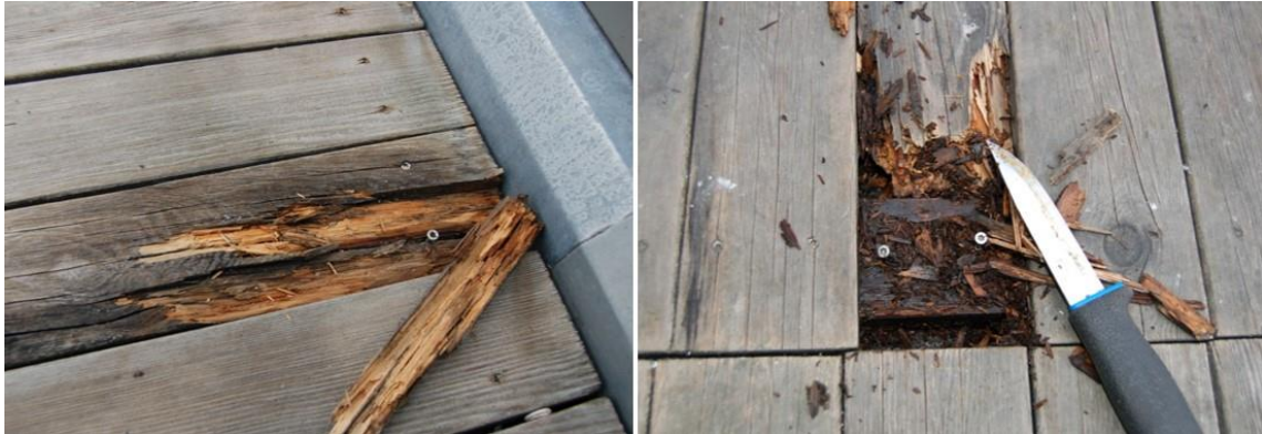
Figure 4: Decay in sapwood region of decking boards of Siberian larch after 6 years in service (Flæte 2016).
